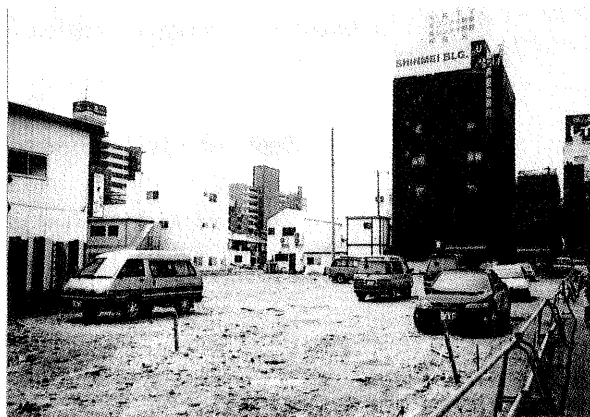
Photograph 1. Fireproof Building (Nagata District)
